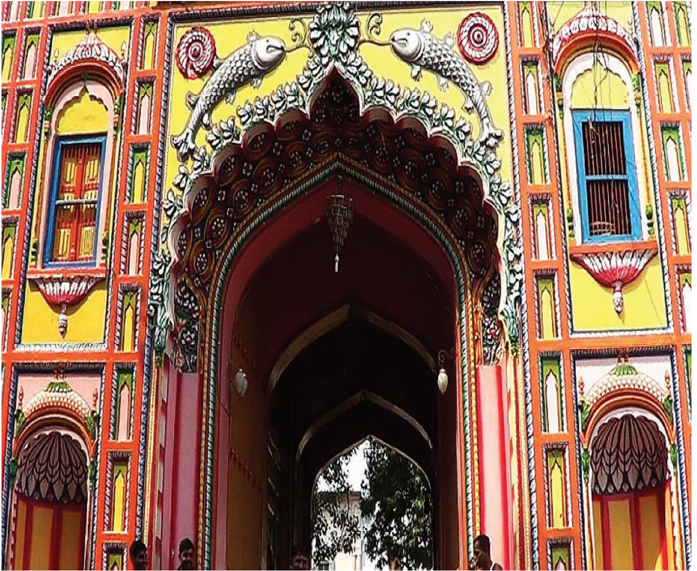
Nageshwarnath Temple entrance
