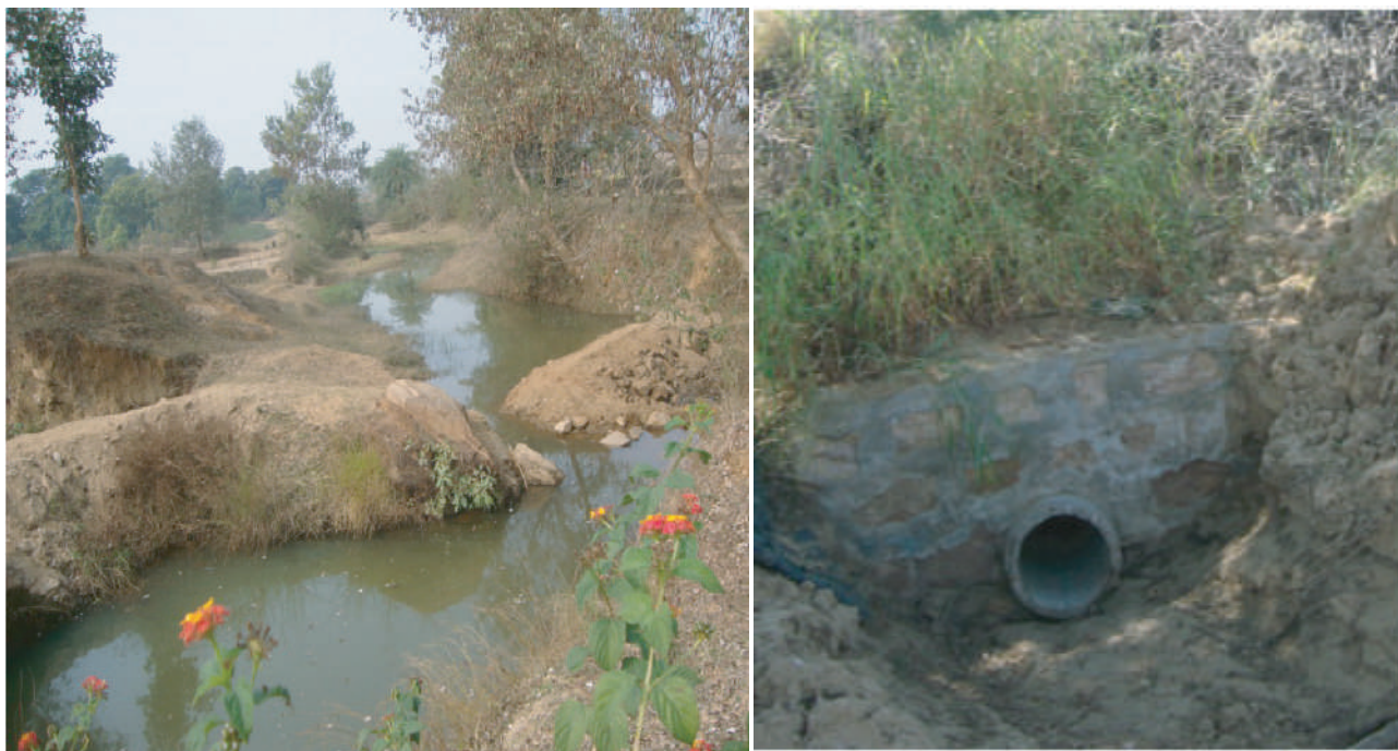
(Left) Water makes its way across rocky channels in Jharkhand; (Right) Paal made of stones to hold water in a khadin The outlet is for the excess water to flow to the neighbouring farm
