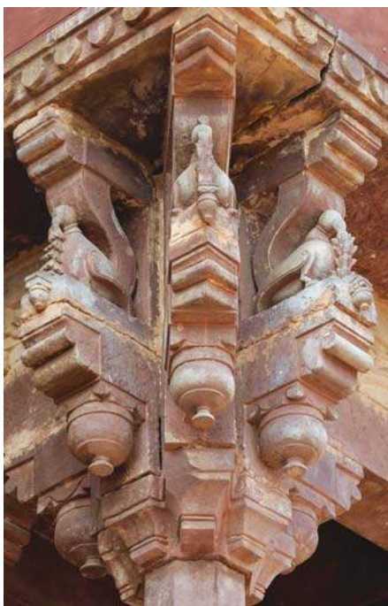
The brackets of a support pillar
