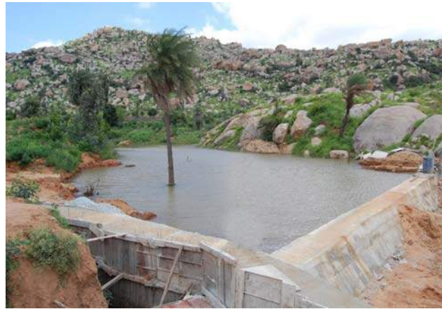
Johads are small earthen check dams that capture and conserve rainwater, improving percolation and groundwater recharge. The last few years have seen a revival of the traditional check dams in Gujarat and Rajasthan.
