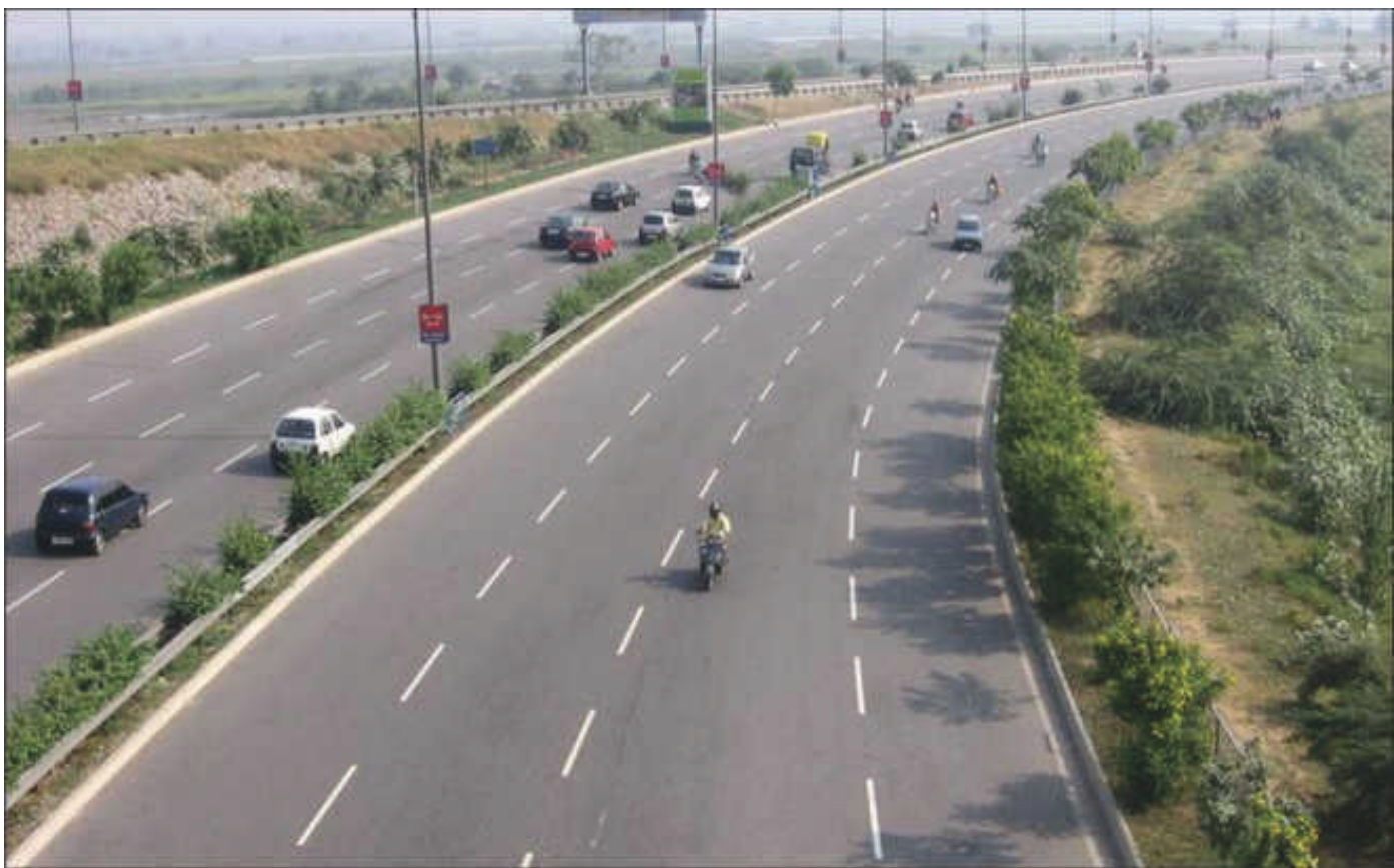
The Kundli – Ghaziabad - Palwal Expressway, a 135 km long and six-lane wide expressway to ease congestion and pollution in the national capital region
