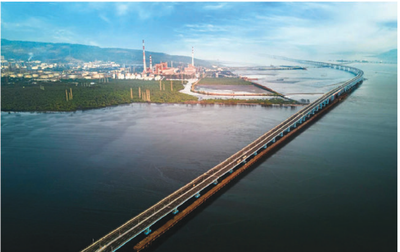
Atal Setu, India's longest sea bridge, an engineering marvel that puts it on par with the world's finest bridges
