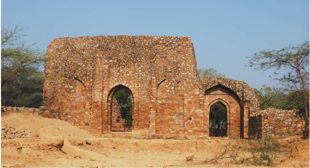
Tomb of Ghiyasuddin Balban, the last ruler of the Slave Dynasty, which contains the first true arch constructed in India
